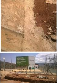
07 Construction of Ketraco Namanga 132/33kv Substation earth works, Equipment Foundation works, Drainage works, Internal Roads, Control Room, Control Room Electrical Installation, Cable trenches, Transformer plinth Foundation, Stone Pitching, Fencing works and ballast spreading.
