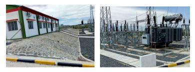
06 Construction of Ketraco Isinya 132/33kv Substation earth works, Equipment Foundation works, Drainage works, Internal Roads, Control Room, Control Room Electrical Installation, Cable trenches, Transformer plinth Foundation, Stone Pitching, Fencing works and ballast spreading.
