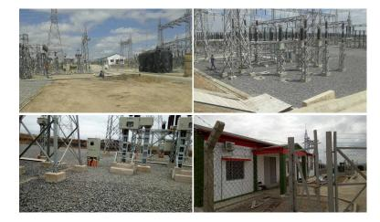
05 Construction of Ketraco Konza 132/33kv Substation earth works, Equipment Foundation works, Drainage works, Internal Roads, Control Room, Control Room Electrical Installation, Cable trenches, Transformer plinth Foundation, Stone Pitching, Fencing works and ballast spreading.
