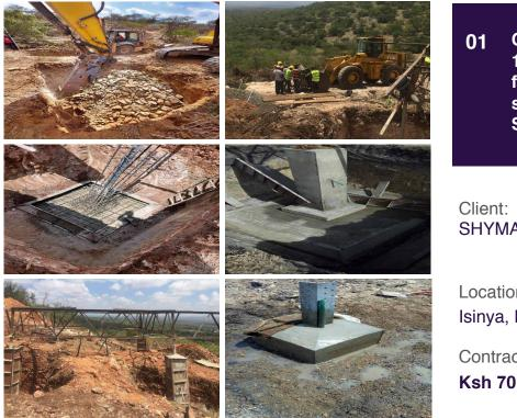
**Construction of KETRACO 132KV Transmission line** foundations from Isinya substation to Namanga Substation.
