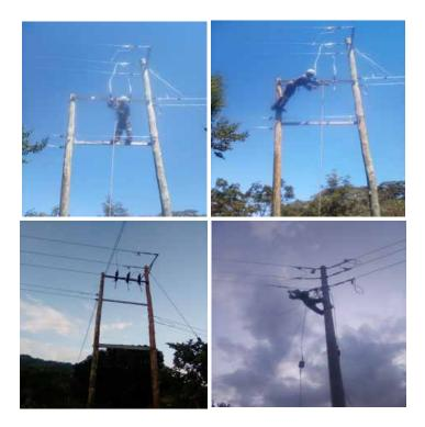
01 Construction of KPLC 33 and 415KV last mile distribution lines in Mwingi county.
